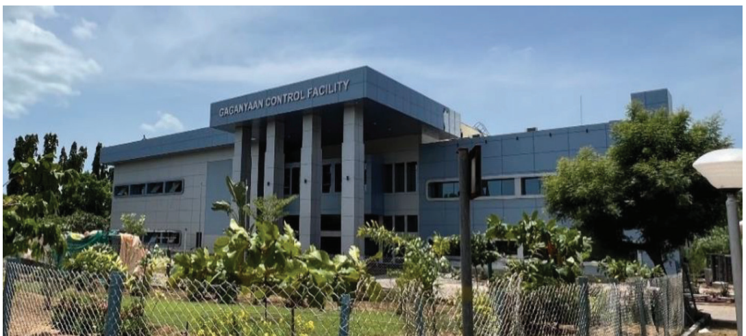
Gaganyaan Control Facility [GCF]
