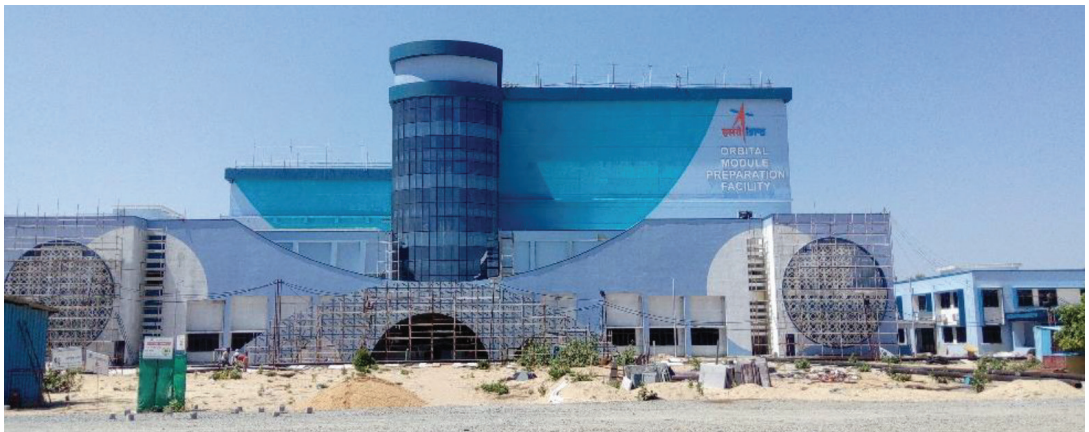
Orbital Module Preparation Facility [OMPF]
