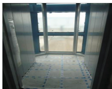
Bubble lift erection at UT
